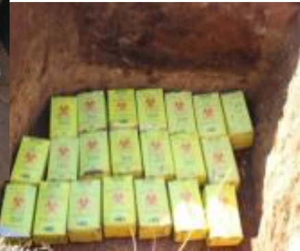
Encapsulation and burial using safety boxes – Madagascar (above) and in concrete drums - Myanmar (right)
