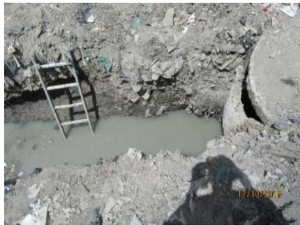
*Image H3c. Possible broken pipe; stagnant water with no flow; possible chemical contamination.*
