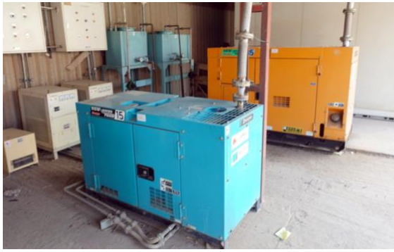
Figure 4. Backup power sources like standby generators should be maintained and tested regularly. There should be enough petrol to cover longest experienced power cut. Power cords of vaccine freezers should be fixed to prevent accidental unplugging.
